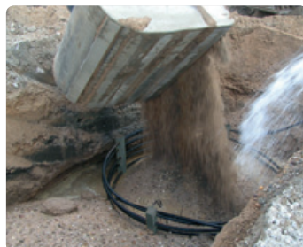
Refilling of the Uponor Energy Cage PE-Xa
