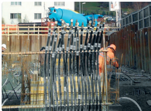
Pressure test of the energy pile installations
