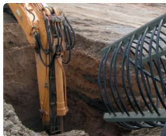
Excavation of the installation pit
