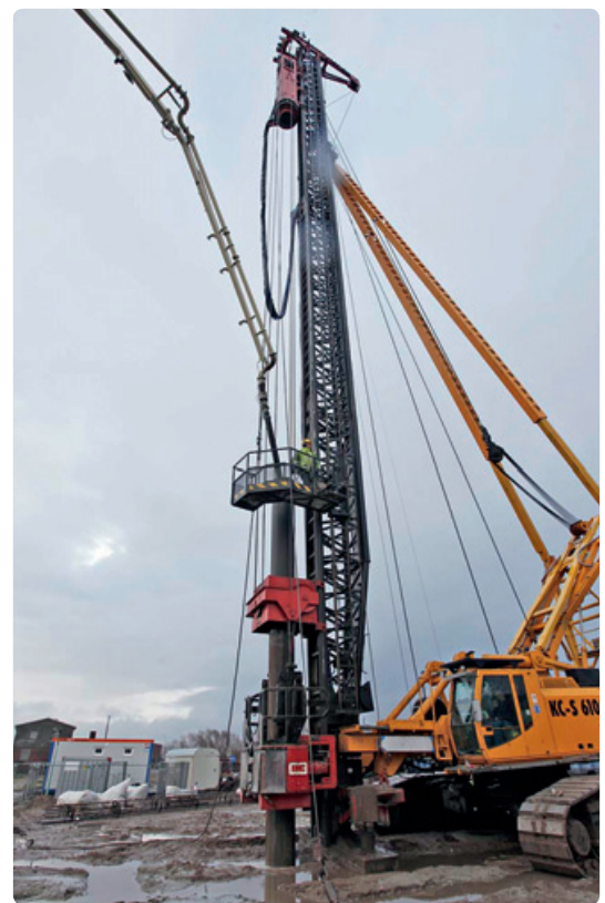
Concreting procedure of the in-situ piles
