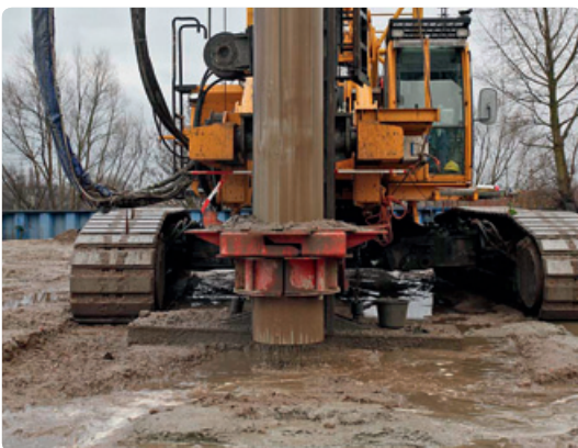
Assembly of a bore pile
