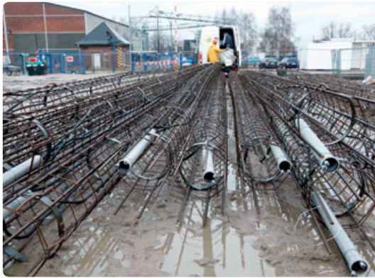
Storage of fitted reinforced cages
