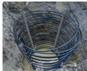
Positioning the energy cage
