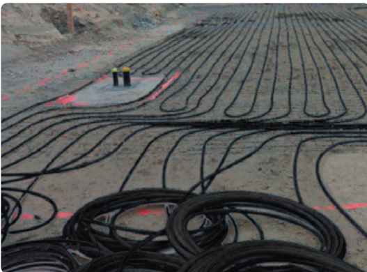
Laying of the individual pipe loops
