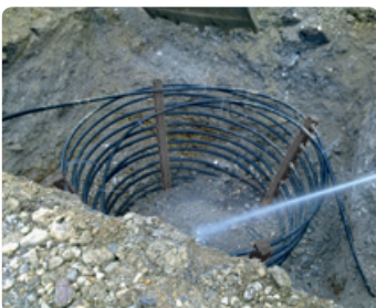
Washing in the filling material
