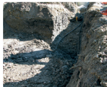
Installed and compacted energy cage
