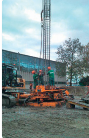
Inserting the steel reinforcing cage in the borehole
