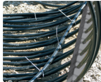
Fixing the return flow line
