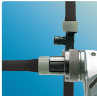
Expanding the pipe end
