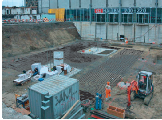
Generation of a floor slab collector
