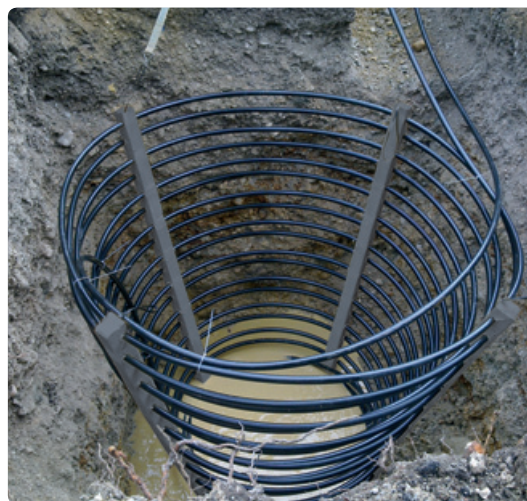
Installation of the Uponor Energy Cage
