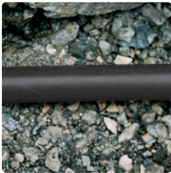
Laying of PE-Xa pipes without sand bed
