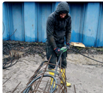
Cutting the inserted pipe loops to length
