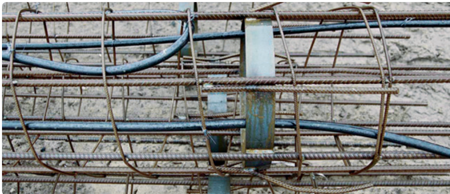
Storage of fitted reinforced cages
