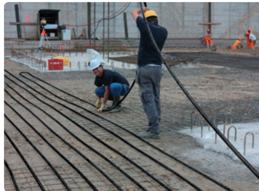
Fixing of the pipe loops on reinforcement mesh
