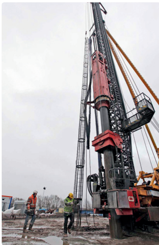
Installing the reinforcing cages
