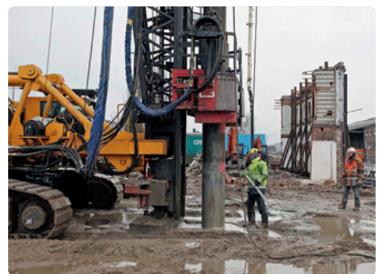
Supervision of the pile assembly
