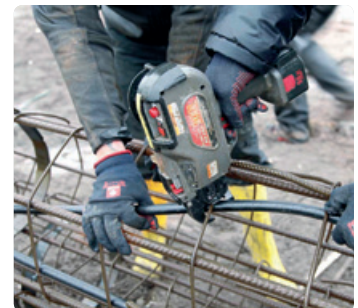
Fixing the pipe loops
