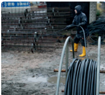
Inserting the PE-Xa pipe loops
