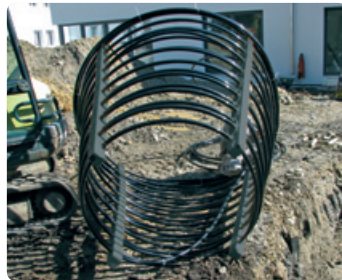
Positioning the connection lines
