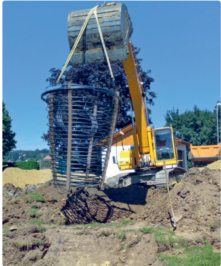
Installation of the energy cage
